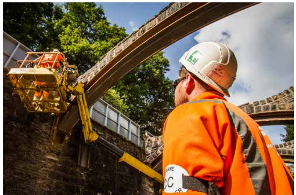
(Below) Adjustments are made to the FRP barrier above the retaining wall.
